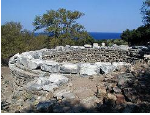
Foundation of the Arsinoë Rotunda and fragment of the dedication (site plan number 15)
